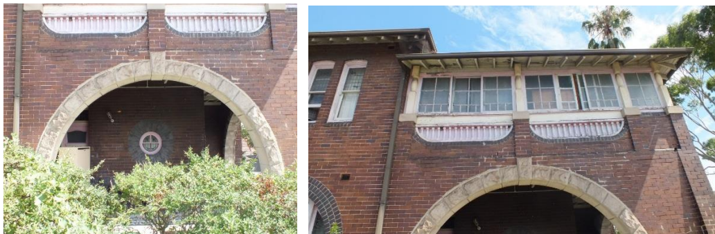
Figure 26 — No 17 Railway Terrace, showing details of stained glass windows, verandah features including turned-timber balustrading and posts (Source: NBRSPARTNERS, January 2015)
