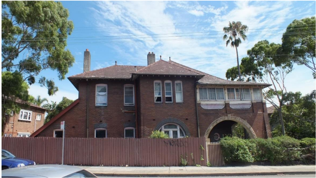
Figure 22 — No 17 Railway Terrace, North Elevation, facing Railway Terrace, showing the timber framed, double-hung sash windows. Slate roof has terracotta ridge and apex ornaments (Source: NBRS+PARTNERS, January 2015)
