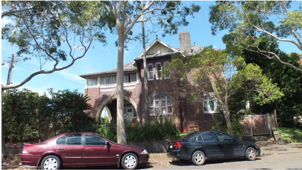
Figure 18 — No 17 Railway Terrace, West Elevation, facing onto Hunter Street, showing the gabled bay with sandstone arches to main entry. The facebrick residence has slate roof, double-hung, timber-framed sash windows are shown on the elevation. No windows contain stained glass. The driveway is located off Hunter Street, to the south of the house (Source: NBRSPARTNERS, January 2015)
