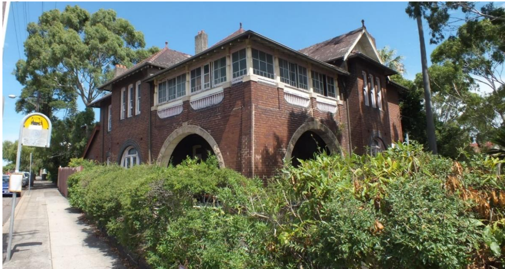
Figure 17 — No 17 Railway Terrace, viewed from the corner of Hunter Street and Railway Terrace. The two-storey, Federation Queen Anne style residence is asymmetrical in design. The facebrick residence has slate roof. The first floor verandah has been infilled with windows (Source: NBRSPARTNERS, January 2015)
