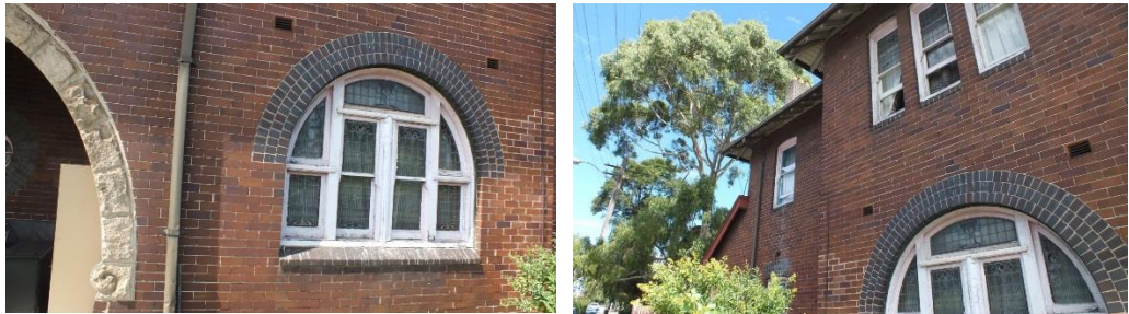
Figure 28 — No 17 Railway Terrace, showing details of original stained glass windows at ground level, contrasting brickwork features around arched windows (Source: NBRSPARTNERS, January 2015)
