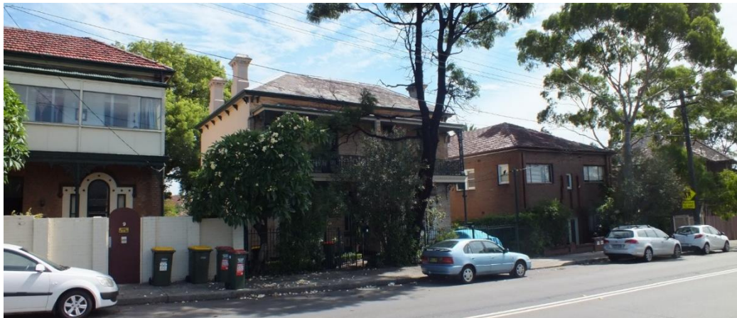
Figure 8 — Two-storey, freestanding residential buildings, Nos 7-15 Railway Terrace, are located on the southern side of Railway Terrace, east of the subject site. The residential buildings date to the Late-Victorian, Federation and Inter-War periods. The masonry buildings have hipped roofs clad in terracotta and slate tiling (Source: NBRS+PARTNERS, January 2015)
