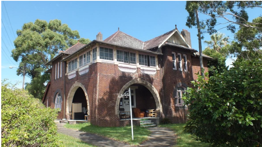
Figure 19 — No 17 Railway Terrace, as seen from the main entry gate at the corner of Railway Terrace and Hunter Street, showing the arched main entry. Original features, including slate roof on hipped and gabled roof structure, rough-cast chimneys, stained glass windows, verandah floor and step tiling (Source: NBRSPARTNERS, January 2015)
