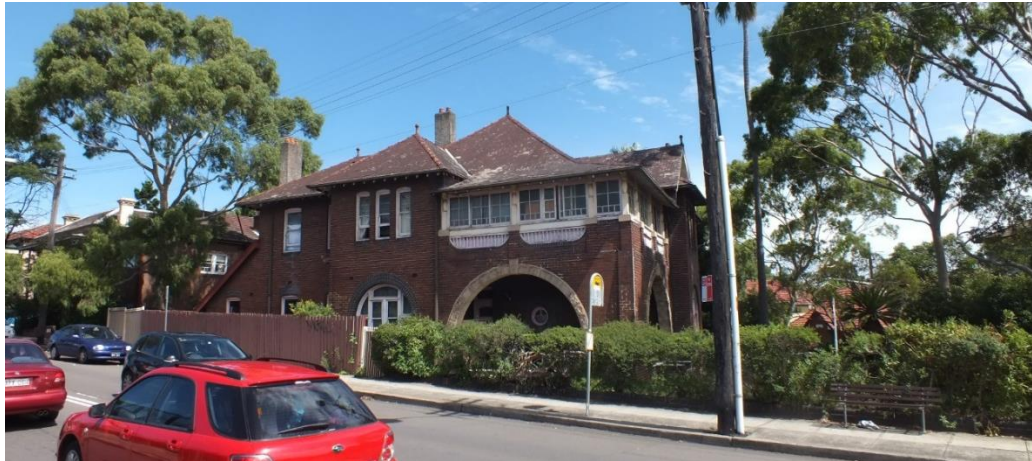
Figure 24 — No 17 Railway Terrace, North Elevation, taken from Railway Terrace, showing the first floor verandah and principal entry (Source: NBRSPARTNERS, January 2015)
