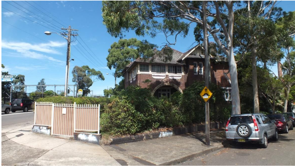
Figure 16 — No 17 Railway Terrace, viewed from the corner of Hunter Street and Railway Terrace. Shrubs located along the perimeter of the residence hide the fencing that has replaced the original boundary markers. A brick upstand is located on the site boundary with fence removed. The later addition aluminium gate is located at the primary entrance on the corner (Source: NBRSPARTNERS, January 2015)
